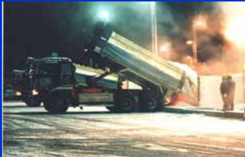
Snow-melting system utilizing residual heat from processed sewerage
