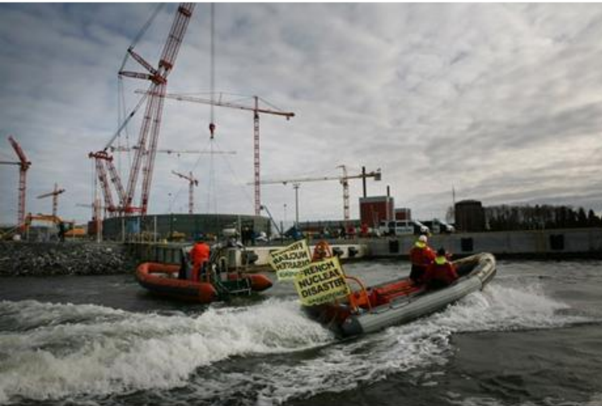
Nuclear Plant Construction
