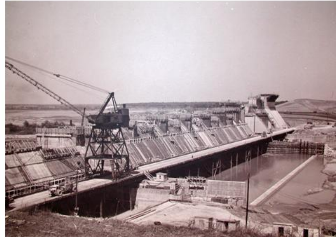
Hydro Electrical Dam Construction
